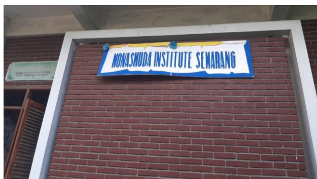
Figure 1. Front view of the Monasmuda Institute Islamic Boarding School
